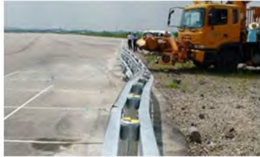
Before installing Safety roller
