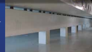
Above: Supporting structures and floor surfaces beneath the electrolysis cells are reliably protected with a polyurethane coating.
