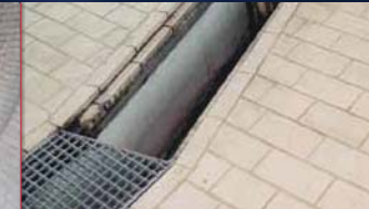
Below: Thermoplastic channels, mechanically anchored in the foundation, with special detailed solutions to connect them up to the tiled industrial floors
