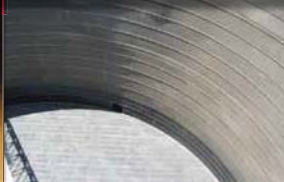
Above: Rubber-lined tank in phosphoric acid production
