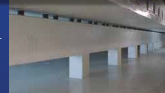
Above: Supporting structures and floor surfaces beneath the electrolysis cells are reliably protected with a polyurethane coating.
