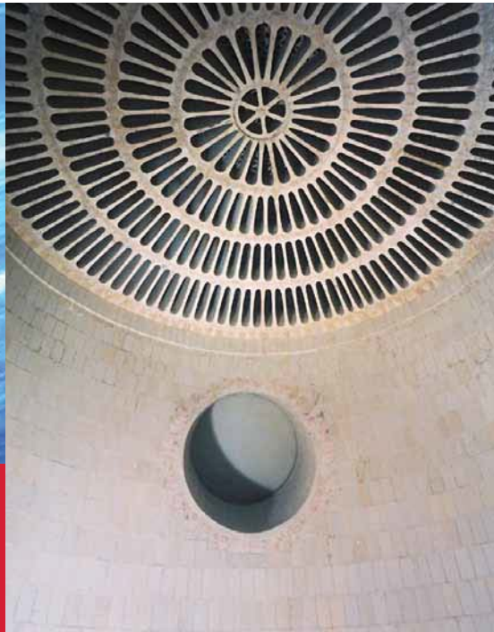
Above: Gas entry pieces and above them a free-standing Steuler Dome, a grid dome made of acid-resistant ceramic material
