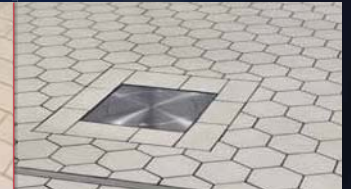
Below: Floors in the pharmaceutical industry are also made to be leak-proof, and with joints
