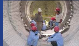
Below: Masonry in autoclaves and flash vessels
