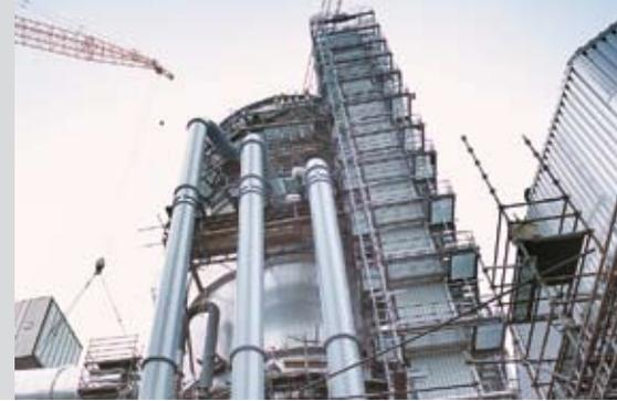
The corrosive sulphur compounds contained in the flue gas place very exacting demands on chemical resistance properties in the scrubbing towers. In addition to the chemical loads, severe mechanical loads are also encountered, particularly as a result of abrasion by finely dispersed solid materials.
