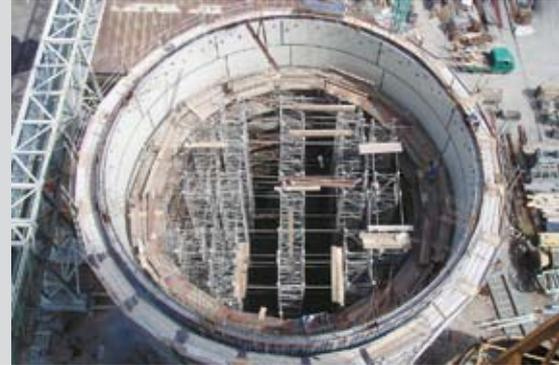
*Photo below: The tank and ceiling construction of the solution tank are completely lined with Bekaplast – smooth surfaces without pores, antiadhesive, highly resistant to chemicals.*
