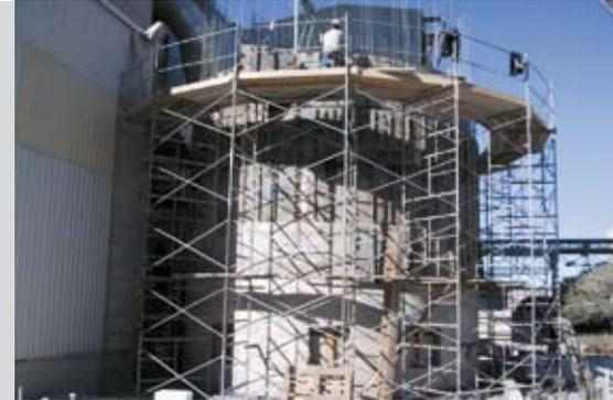
Thanks to its outstanding chemical, thermal and mechanical resistance properties as well as its exceptionally high resistance to abrasion, polypropylene is also employed as a mechanically anchored corrosion protection lining in concrete scrubber constructions.
