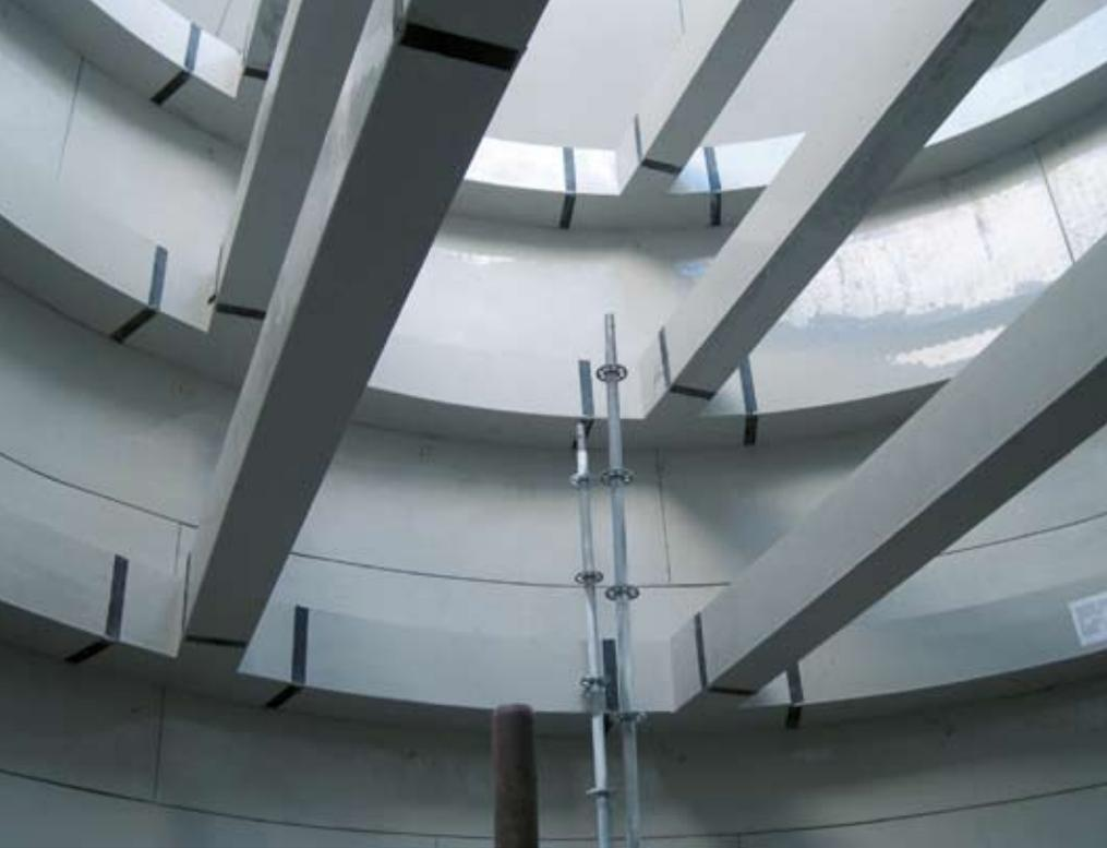
Photo on the left: Concrete girder construction, lined with Bekaplast, designed to support the mist eliminators.
