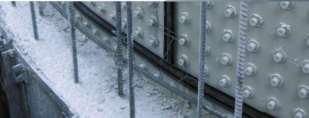
Photo on the left: The Bekaplast sheets are mounted onto the inner formwork for the concreting operation the individual sheets are still interconnected by means of special sealing strips.
