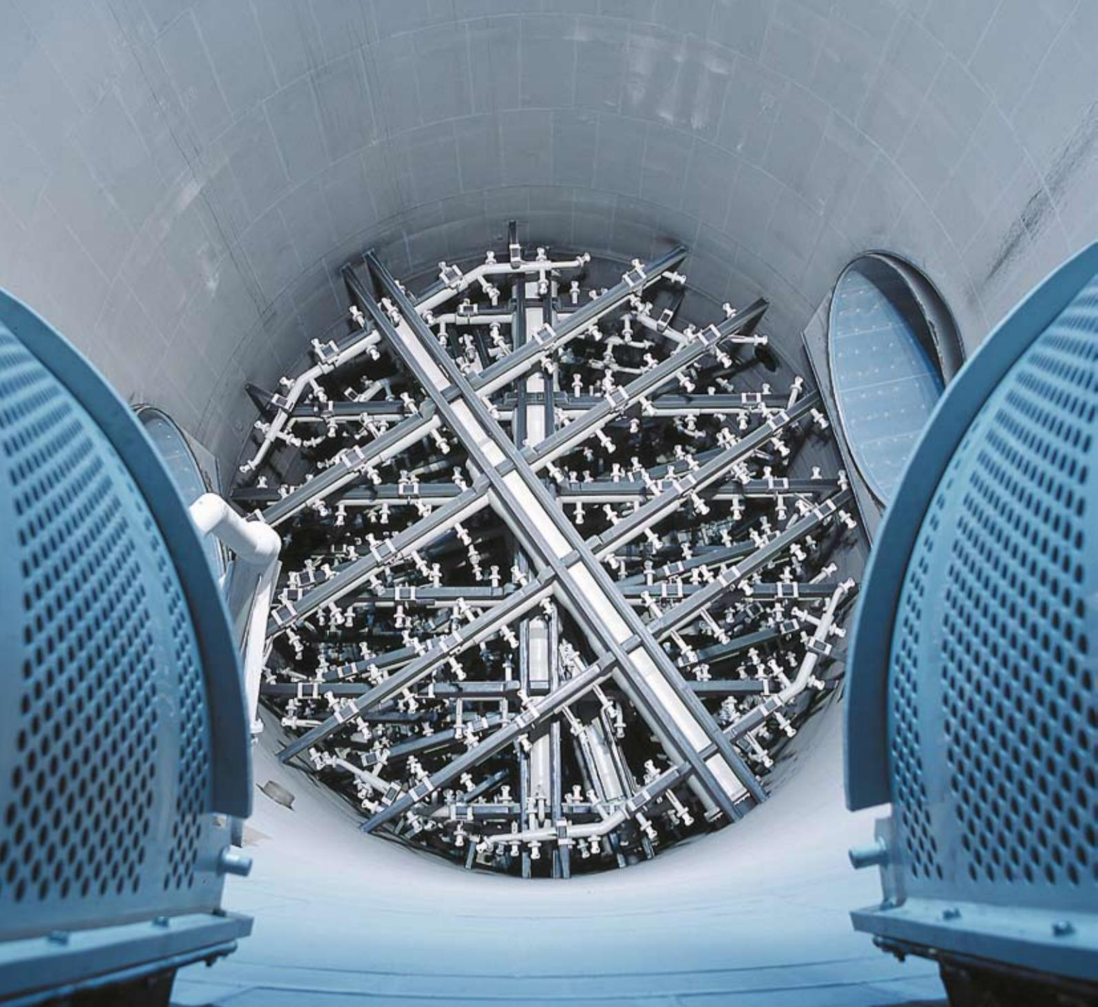
Modernisation measures in a brown coal-fired power plant: Steuler was awarded the contract for the execution of the design, manufacture and assembly of the spray piping systems for the scrubber of the new flue gas desulphurisation plant.
