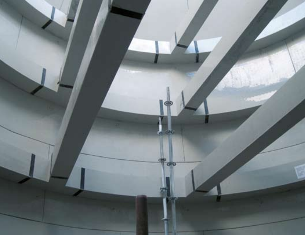
Photo on the right: Concrete scrubber construction with mechanically anchored polypropylene lining and spray levels. The thermoplastic sheets are welded together to ensure a gas- and water-tight assembly. This process guarantees the execution of a testable, homogeneously lined chamber that is resistant to severe chemical, thermal and mechanical loads.
