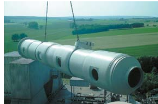
Photo above: Often there is only a very narrow aperture through which the spray pipes have to be installed. To facilitate their installation, Steuler manufactures all distribution pipes in pre-determined segment lengths.
