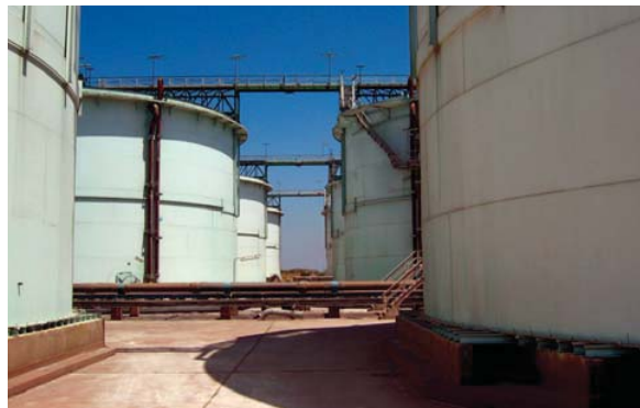
Above: Coated storage tanks in the fertiliser industry.
