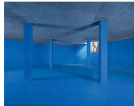
Above: BEKAPLAST™ Lining 400 lined drinking water tank.
