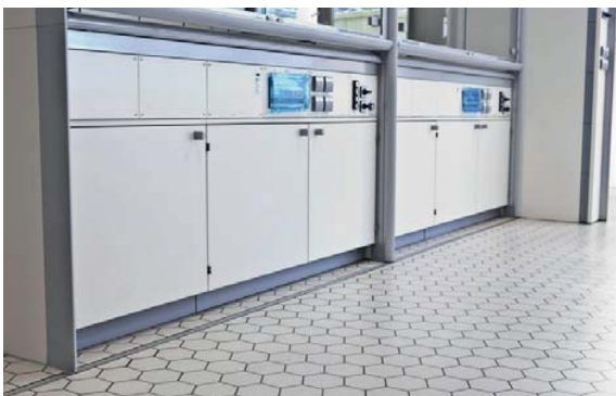
Above: Ceramic tiles are laid on chemically resistant sealing layers using equally resistant synthetic resin mortar and grouting.
