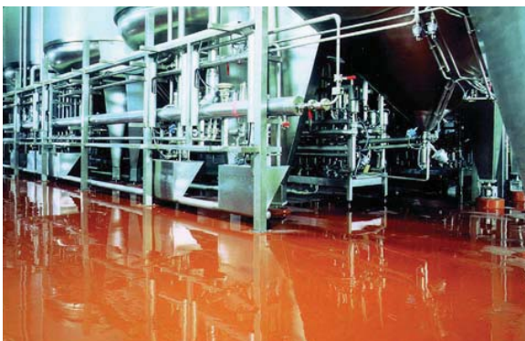
Above: Self-levelling industrial flooring in the food industry.
