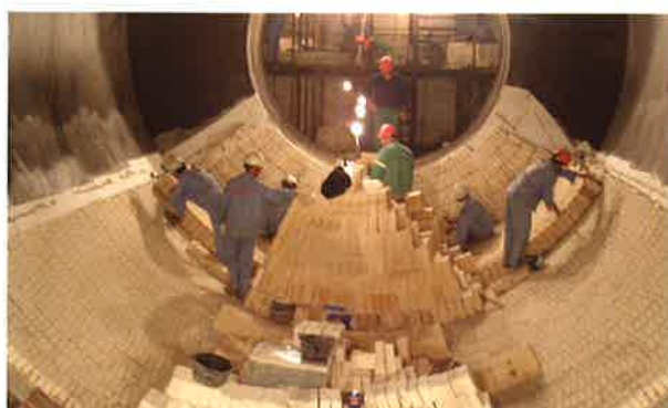
Multi-layered brick lining of a sulphuric acid cracking plant
