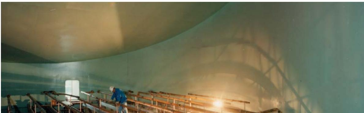
Above: Coated absorber head in a flue gas scrubber plant.
