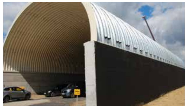
Fig. 9. Placement of the ribs in longitudinal direction of the structure
