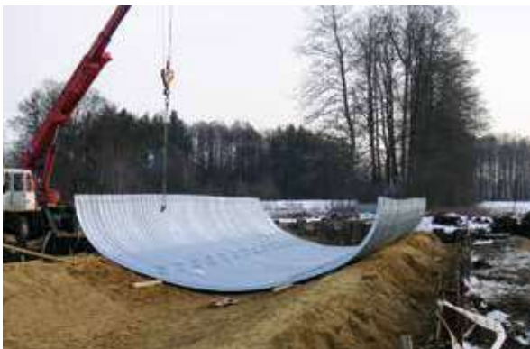
Fig. 11. Connection of SuperCor® structure with flexible footing
