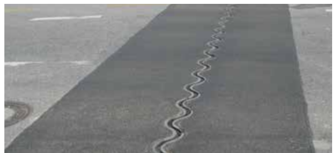
MAURER Low-Noise Single Seal Joint
