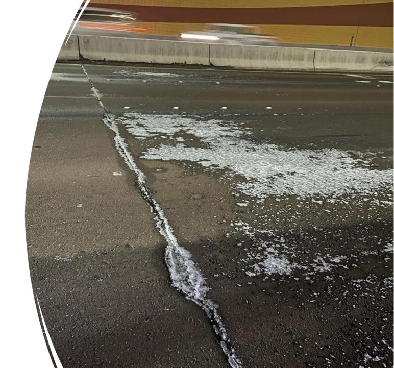
Injection can cause damage to the waterproofing if executed without considering the waterstop pressure limitations.
