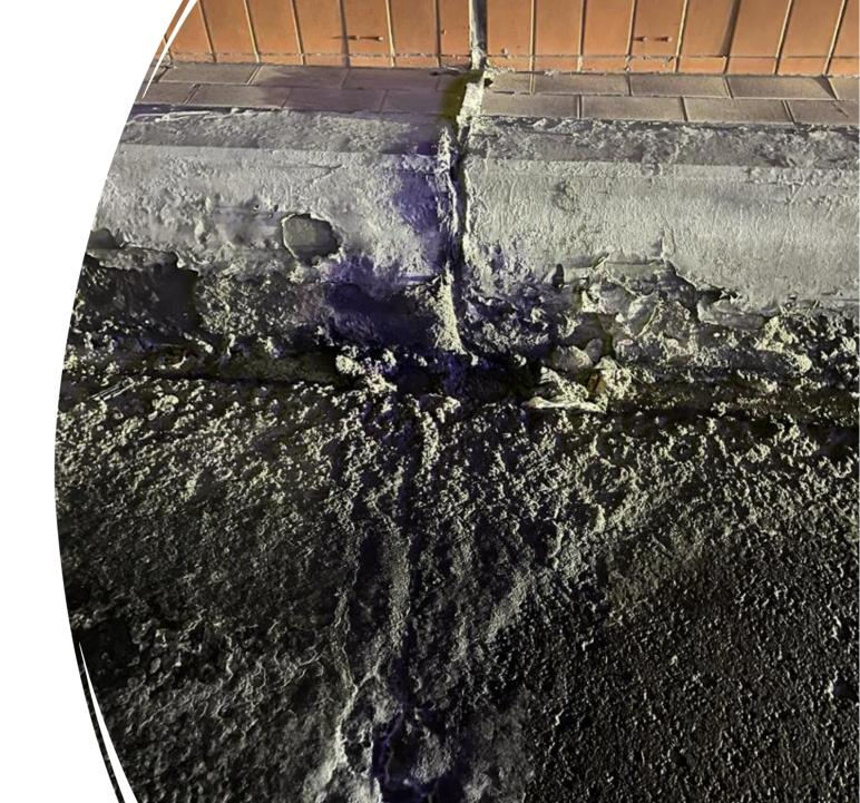
Not only between joints, also middle of the road are showing leaks.
