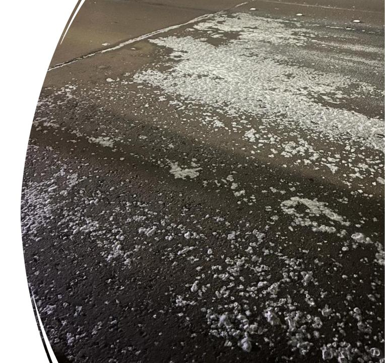
High concentrations of salt may cause long term damage to concrete and reinforcement which will affect the integrity of the structure.
