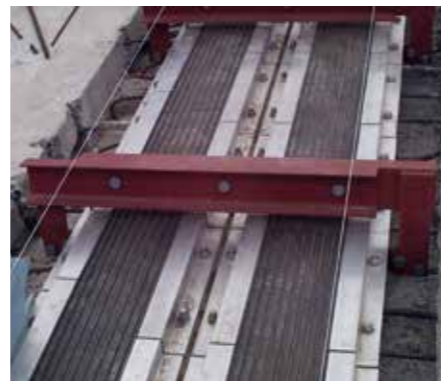
Installation of MAURER Double Mat Joints
