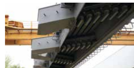
Craned MAURER Swivel Joist Modular Joint
