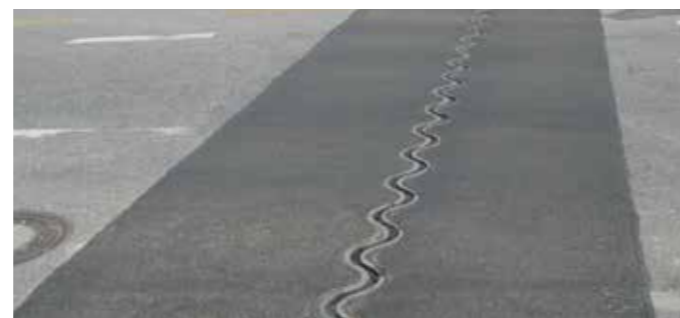
MAURER Low-Noise Single Seal Joint
