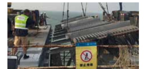
Inserting MAURER Sliding Lamella Joints into the structure
