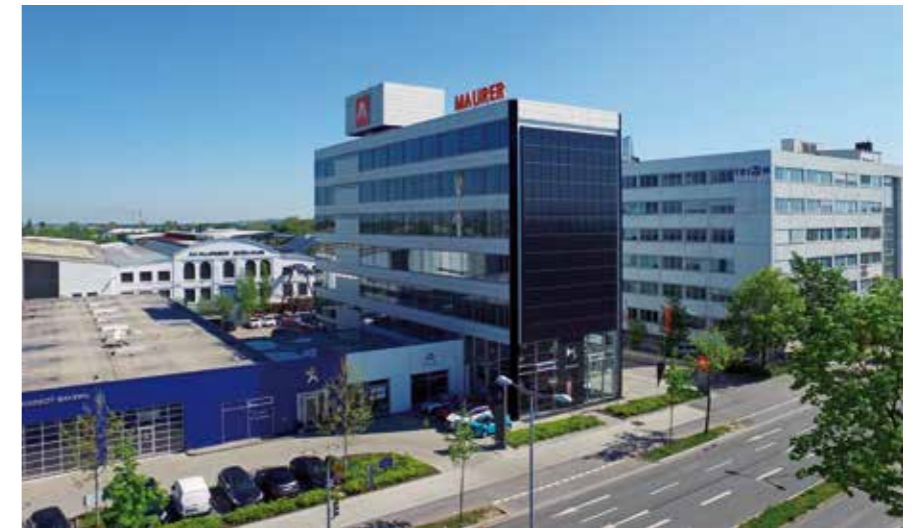
MAURER headquarters, Munich / Germany
