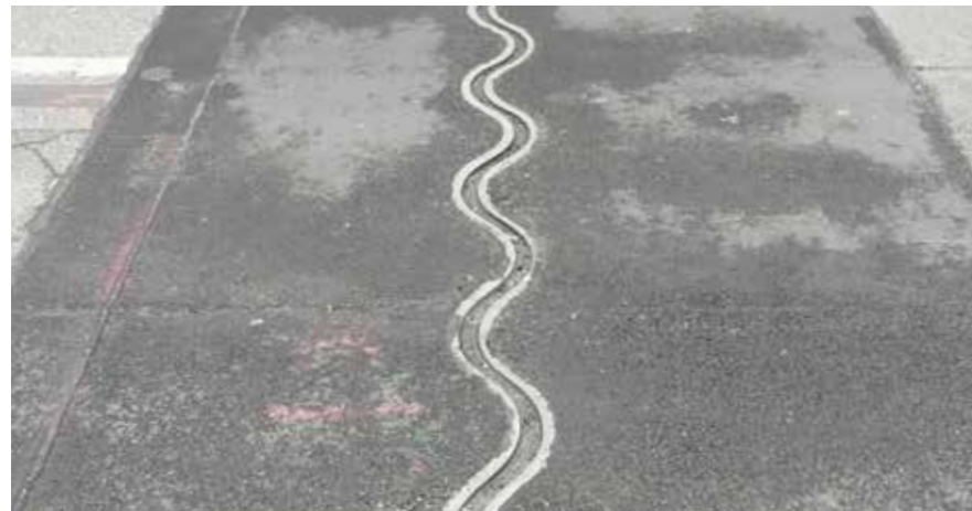
Donnersberger Bridge, Munich / Germany
